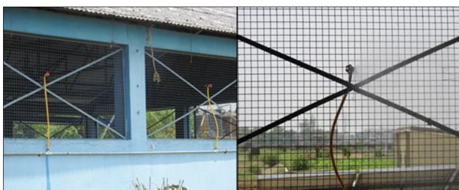
Fig 6: Installation of nozzles in cattle barn
