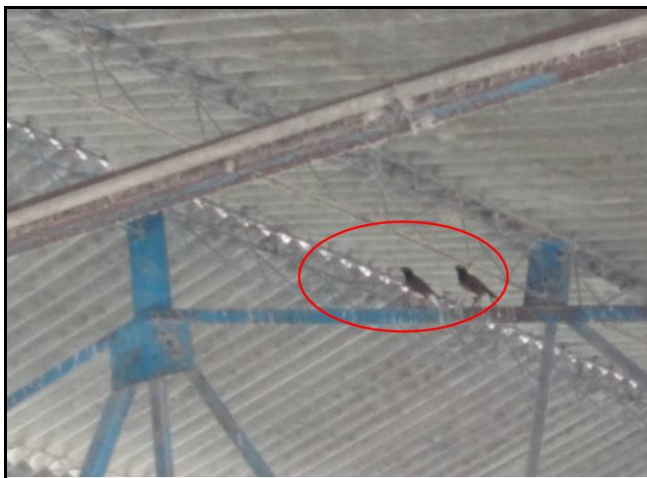
Plate 1.2: A pair of myna perching on the truss
