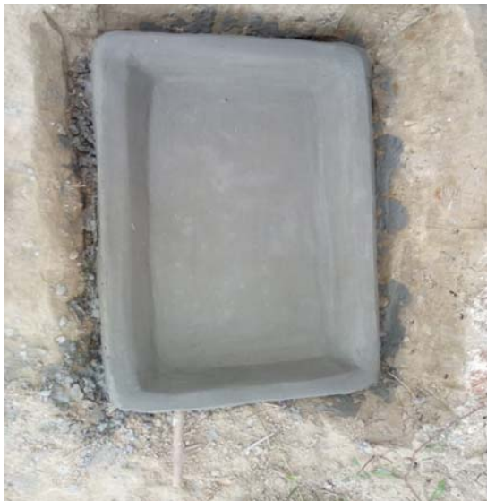
Fig 1: Newly Constructed Foot Bath
