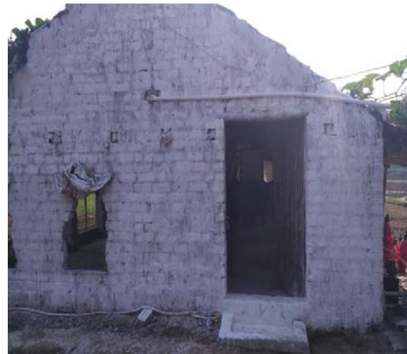
Fig 4: White washing outside walls of the shed
