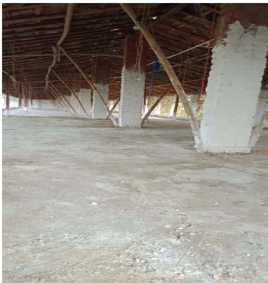
Fig 2: Completed white washing inside view
